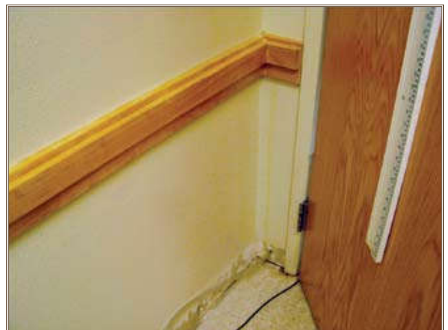
After the room was treated with the hydrogen peroxide gas process, the same wall shows the mold and mildew have been eliminated.
