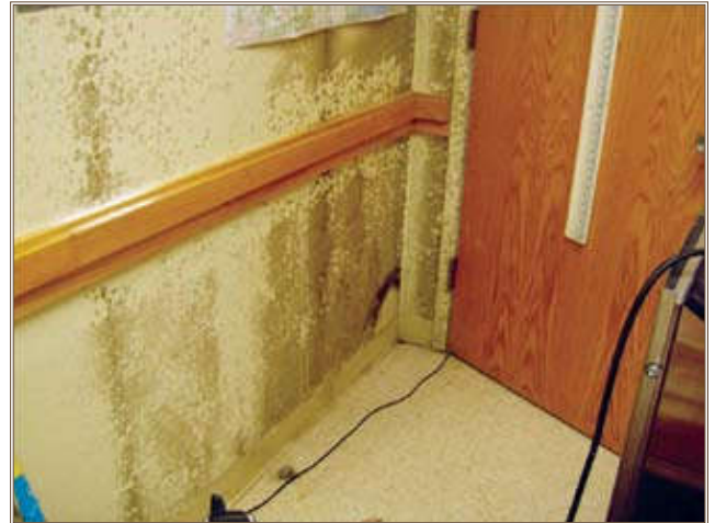
Before treatment, this barracks room wall is covered with mold. Photos courtesy of Pat Fields
